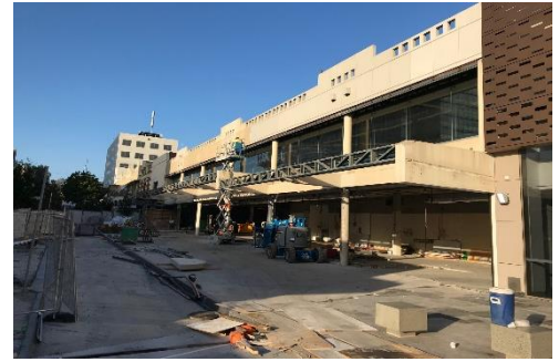
Demolition works of the awning
