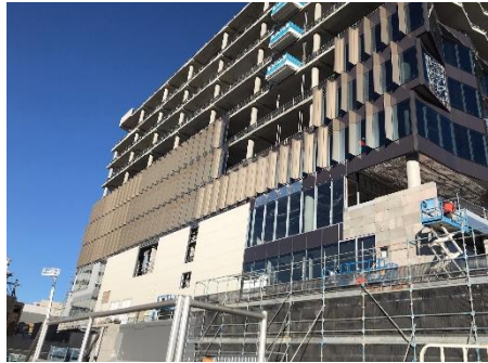
Administration building stone façade and curtain wall
